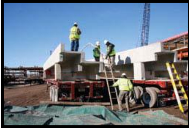
Figure 101: Precast Members Being Delivered - (Sawyer)
