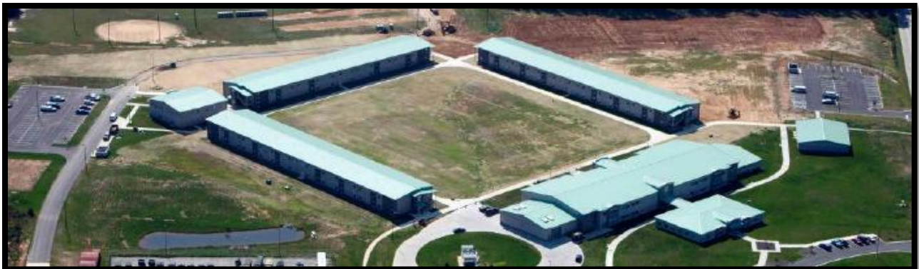
Figure 2: RTI Campus - Courtesy of Barton Malow
