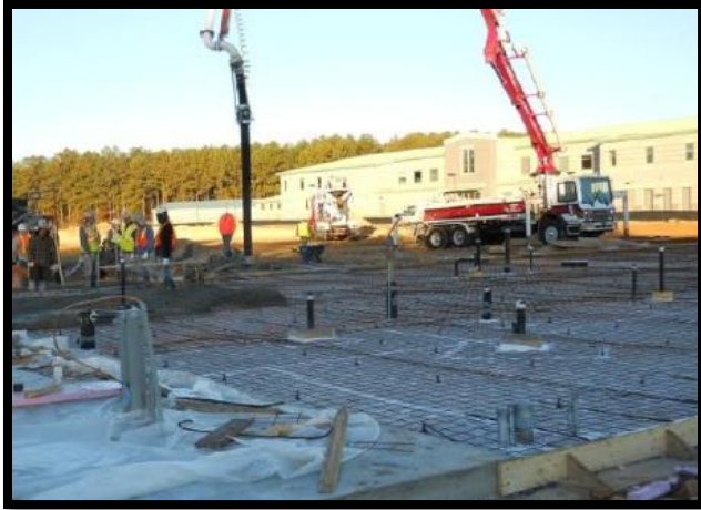
Figure 14: Slab on Grade - Courtesy of Barton Malow
