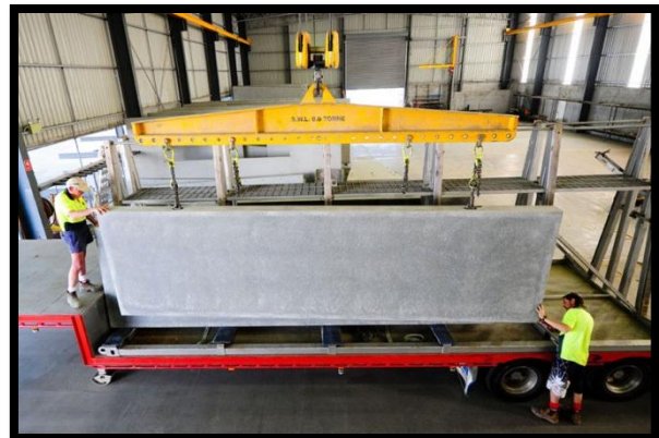
Figure 90: Panels Being Placed on Truck Bed (“Gate Precast”)
