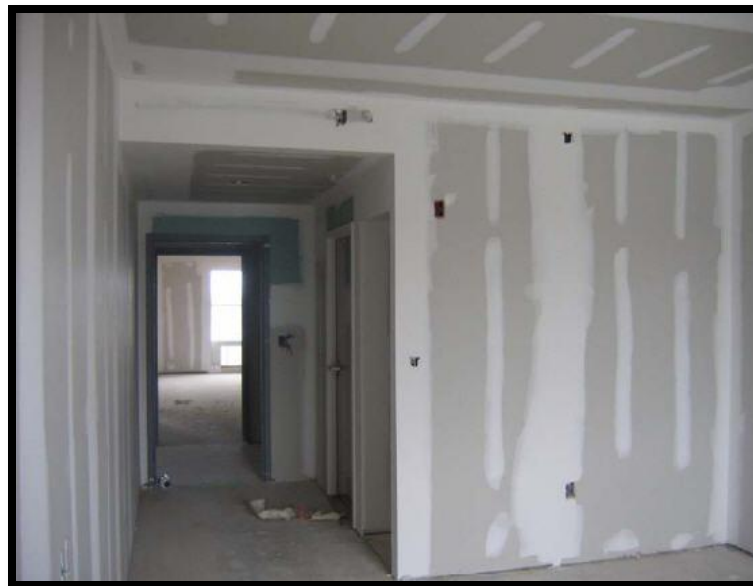
Figure 44: Framing the Pods into the Building (Mensch)
