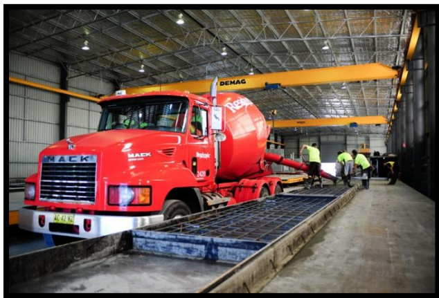
Figure 88: Concrete Delivery (“Gate Precast”)
