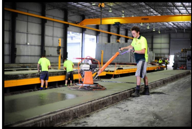
Figure 89: Working Environment (“Gate Precast”)
